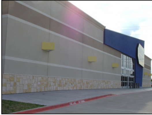
Figure 3: Building without Foundation Plantings
