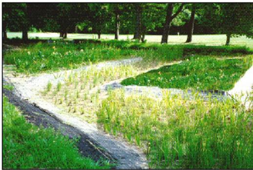
Newly Constructed Shallow Wetland
