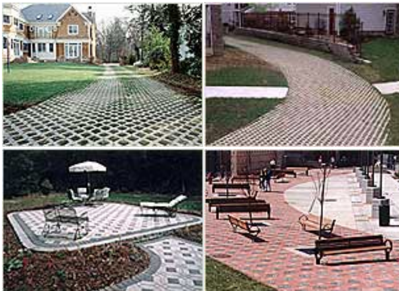
Figure 24.4 Examples of Porous Paver Surfaces
