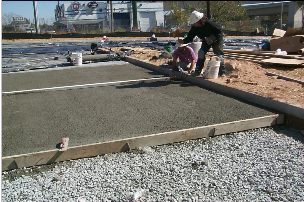
Figure 25.2 Porous Concrete System Installation
