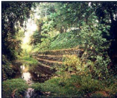
Figure 3.22 Gabion Baskets Installed for Slope Stabilization along a Stream
