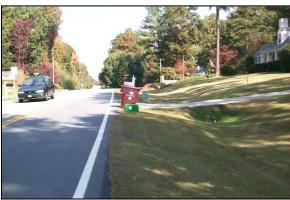
Figure 2.31 Using Vegetated Swales Instead of Curb and Gutter
