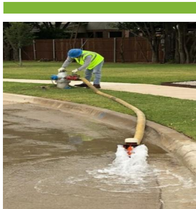
Flushed dead end lines 500 times
