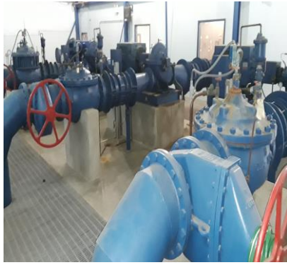
2 Water Pump Stations Repaired
