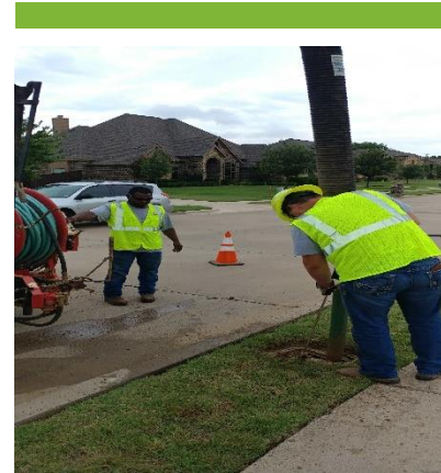
150 Meter Box Replaced & 75 Meter Sets
