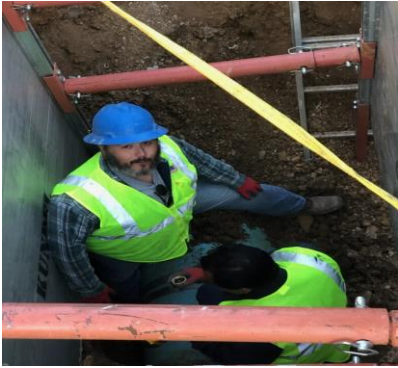
10 Water Main Repairs
