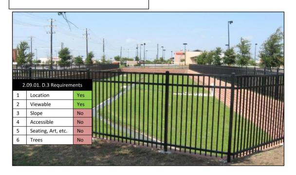
Figure 5: Example of a Detention/Retention Pond not Designed as an Amenity
