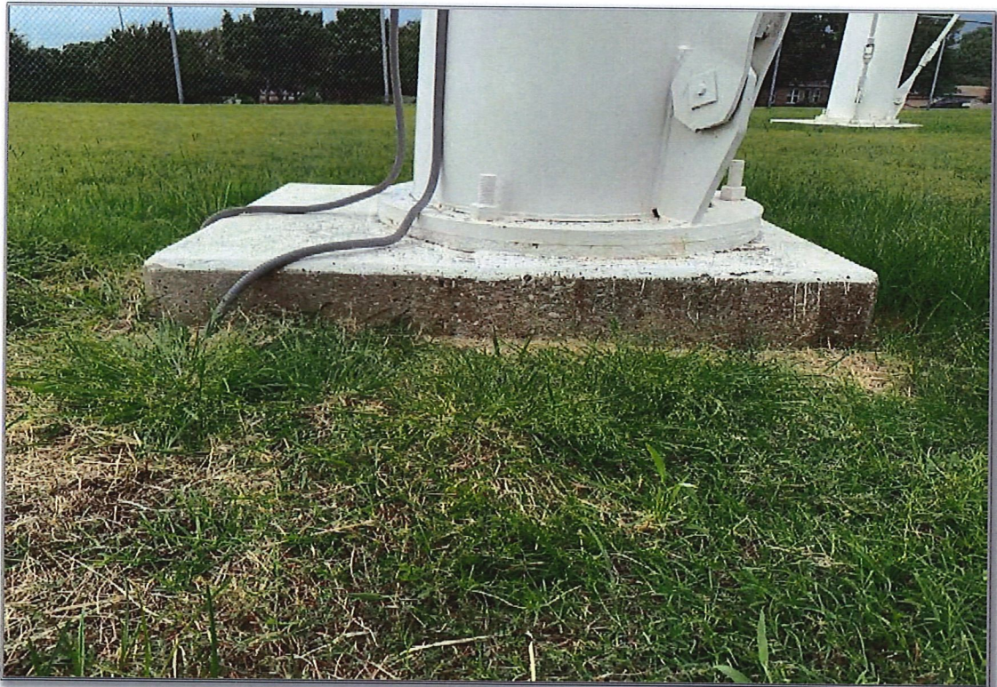
8) TOWER LEG AT GROUND SURFACE
