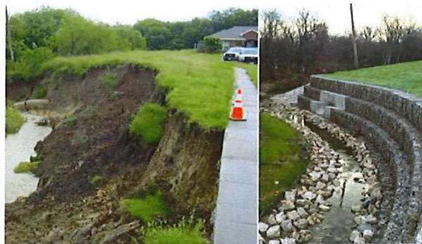
An eroded channel is restored using a gabion wall and rock riprap within the channel.
