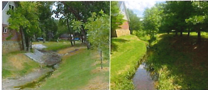
Left: A gabion mattress and turf-reinforcement matting, shown shortly after construction, help protect a garage against stream channel erosion. Right: Fifteen years following construction, the channel's integrity has remained intact
