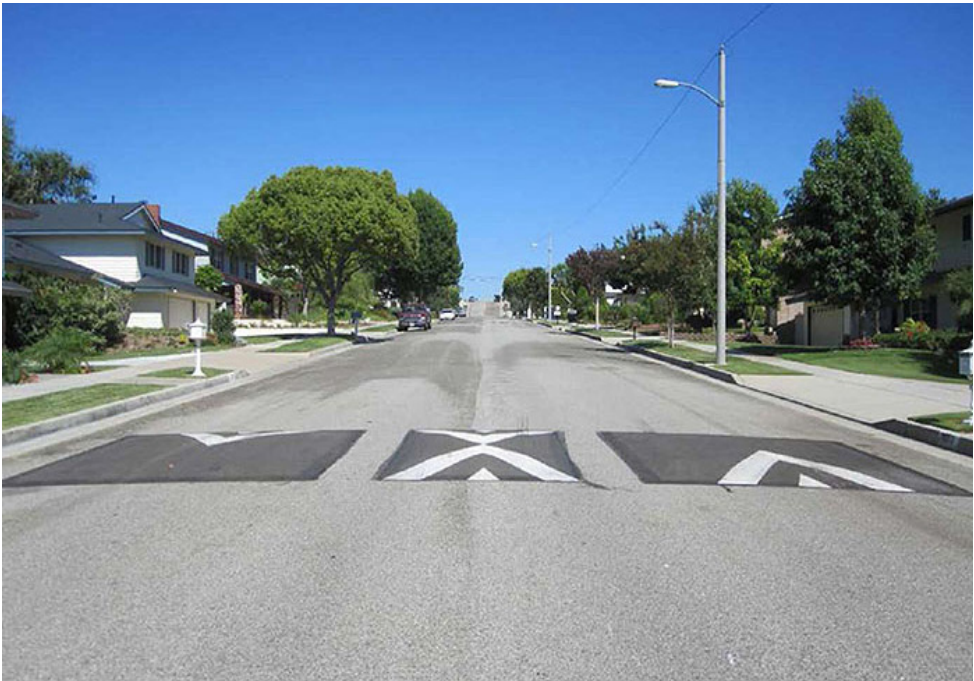
Speed cushions with passage that straddles centerline. (Credit: Jeff Gulden)
